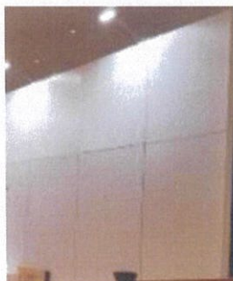
EXAMPLE of NOT ACCEPTED: modular system with visible joint elements
